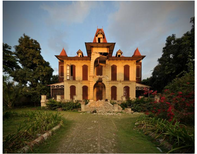
Fig 11 A late 19 th century house in Port-au-Prince after the 2010 earthquake. The construction of the masonry walls in this house is a combination of brick and rubble stone. Despite the use of extensive internal sections of rubble stone, the house remained standing, although extensively damaged – thus showing a better performance than at least 40% of the reinforced concrete buildings in Port-au-Prince, which collapsed.
