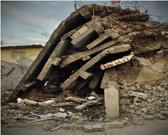
Fig.9 Remains of a collapsed multi-storey building in Port-au-Prince Haiti after the 2010 earthquake that devastated the city. The pancake collapse of reinforced concrete buildings is usually lethal to most of the occupants, and because of the strength of the concrete floor slabs, the finding and extraction of the survivors in time is exceedingly difficult.
