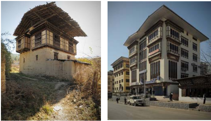
Fig 13 A comparison of a traditional rural Bhutanese house of rammed earth and timber construction ( left ) next to a new hotel in downtown Thimphu of reinforced concrete frame construction. The traditional rabsel , or projecting window-wall can be found on both buildings, but it appears tacked onto the side of the modern structure, rather than an integrated and culturally consistent part of its architecture. [4]
