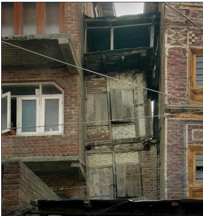
Fig. 14 A view in 2005 of a traditional building in Srinagar, Kashmir where part has been demolished and replaced with a new concrete block, probably after the building was subdivided between two members of the same family.
