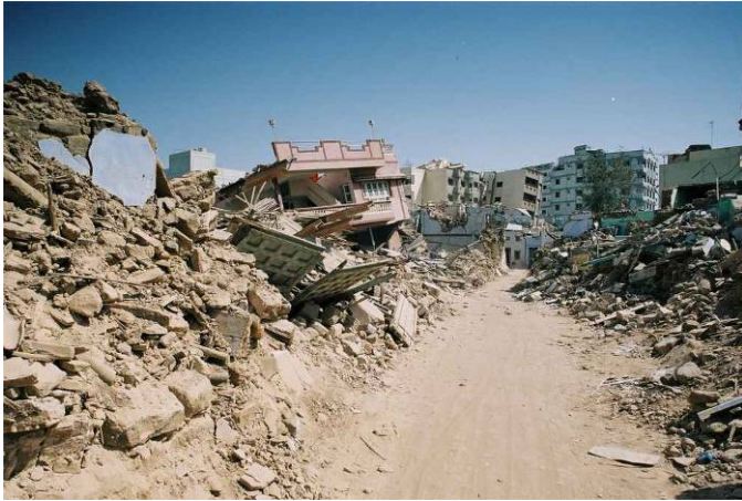
Fig. 3 A view within the historic walled city area of Bhuj after the 2001 Gujarat earthquake. In this area of the city, most of the historic buildings were of rubble stone masonry construction and the modern buildings were of reinforced concrete. As can be seen in the photograph, the earthquake destroyed many of both types of construction.
