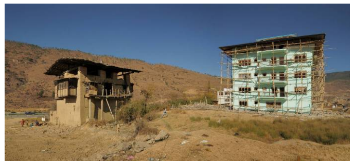
Fig 12 A traditional rammed earth and timber Bhutanese house on the edge of Thimphu next to a new multi-story house of reinforced concrete construction. [4]
