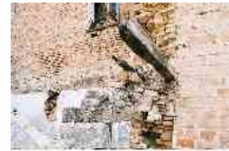
View of masonry house in Ahmedabad showing the timber beam that had been imbedded in the mortar.
