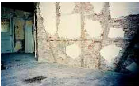
Damaged "Hımsı" house in Düzce showing intact infill wall under plaster shed by the "working" of the wall
