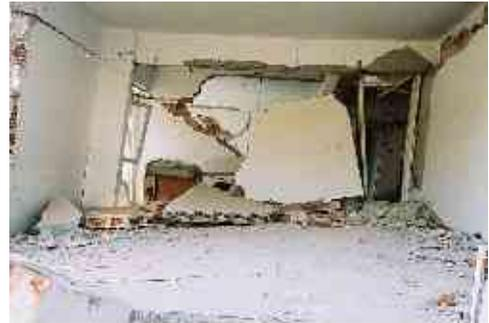
RC construction in Golcuk after earthquake showing collapsed infill wall.
