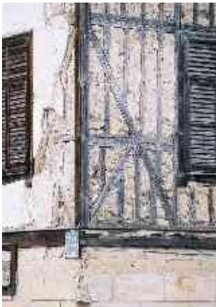
"Hınıs" house with stone infill with mud and lime mortar, Saffronbolu
