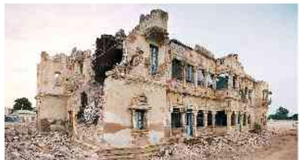
Bhuj Hospital, a masonry building without timber lacing, showing effects of the earthquake
