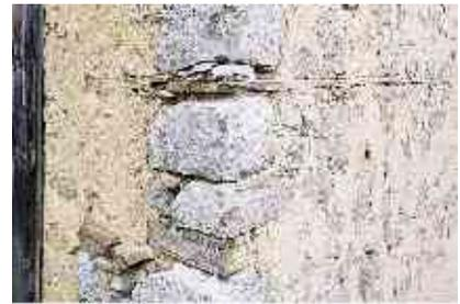
Detail of stone 1st story of house showing "*hatıllar*" imbedded in wall, lapping at the corners.
