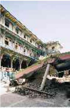
Swaminarayan Temple showing its infill frame building surviving with very little damage behind a portion of its reinforced concrete addition that collapsed. Bhuj
