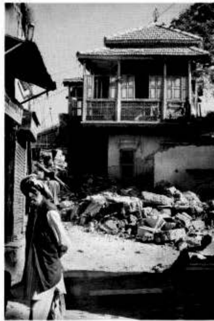
Fig. 12. This house has survived at least the most recent two major earthquakes that otherwise devastated Anjar’s old town center. The balconies on two walls helped to keep this house standing while most buildings around it fell.
