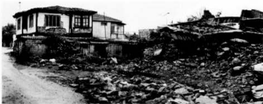
Fig. 1. A timber and masonry house in Adapazari, Turkey, remains standing, having lost only its stucco, next to a collapsed reinforced-concrete apartment house. All photographs © the author.
