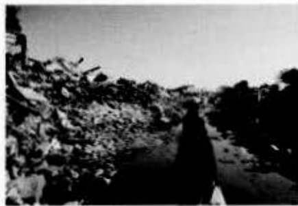
Fig. 11. The ruins of Anjar town center in western Gujarat, India, a month after the earthquake.
