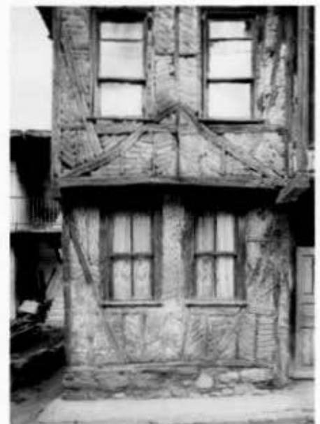
Fig. 5. This house was constructed in 1955 by the father of the two brothers who currently live there with their families. It survived with only cracks in the interior plaster just a few blocks away from rows of new reinforced-concrete apartment houses that collapsed.
