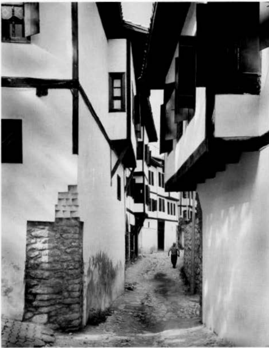
Fig. 4. Street with overhanging jetties, in Safranbolu, Turkey. The cantilever of the upper story over the lower story helps to hold the masonry walls together. The timber lacing is hidden by the plastered surface.
