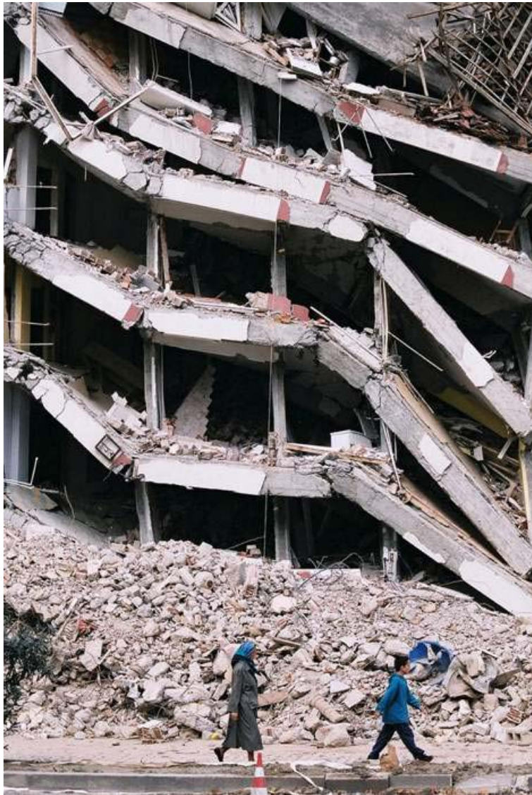
Figure 15: Collapsed Reinforced concrete building in Gölcük.
