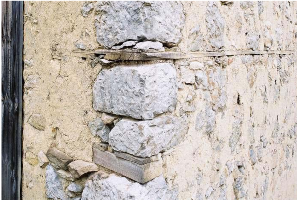
Figure 10: Laced bearing wall in Safranbolu, Turkey
