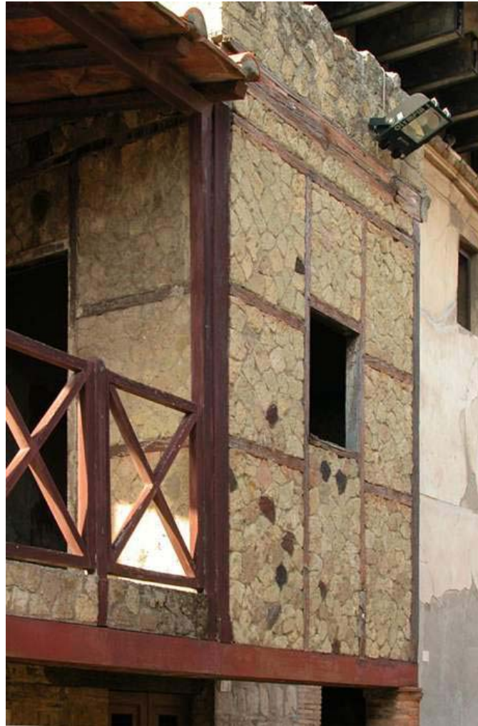
Figure 3: Pre-79AD Infill-frame construction found and restored at Herculaneum.
