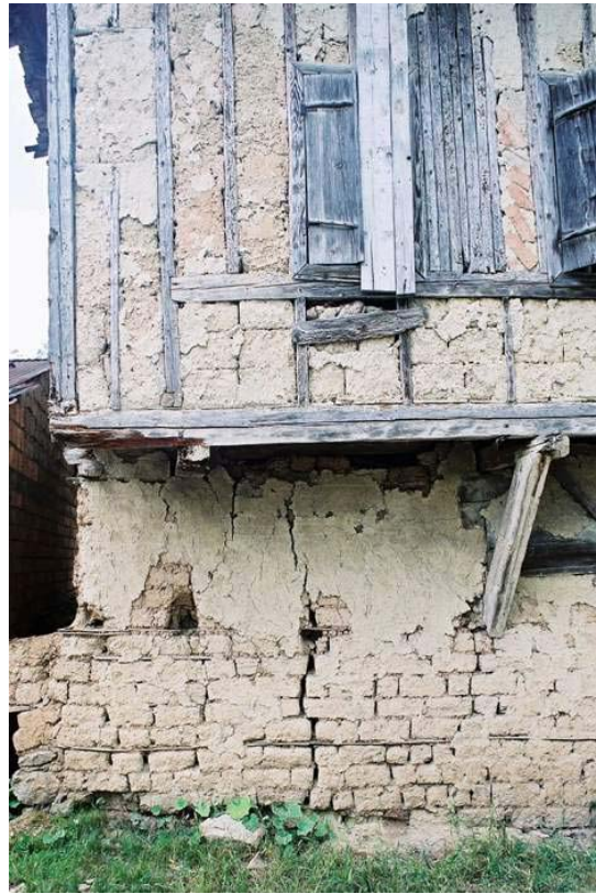
Figure 4: View of Infill-frame construction in the historic Ottoman town of Safranbolu, Turkey
