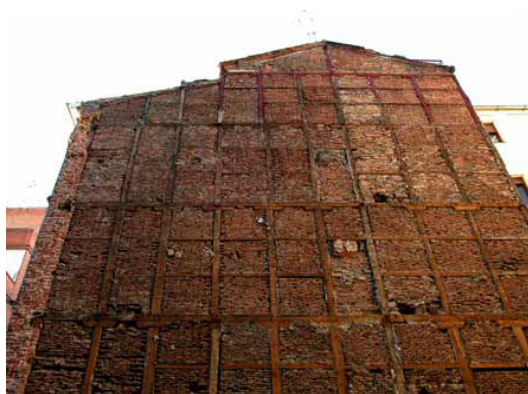
Figure 16: Pombalino “Gaiola” walls in Baixa, Lisbon, Portugal.
