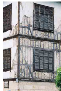
Figure 3: Large 3 story house in himiş construction, Safranbolu, Turkey, 2000.
