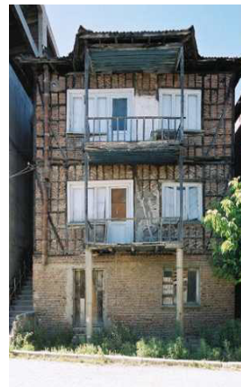
Figure 5: Row of collapsed RC buildings showing typical hollow clay block infill on end wall left exposed by the collapse of another building.
