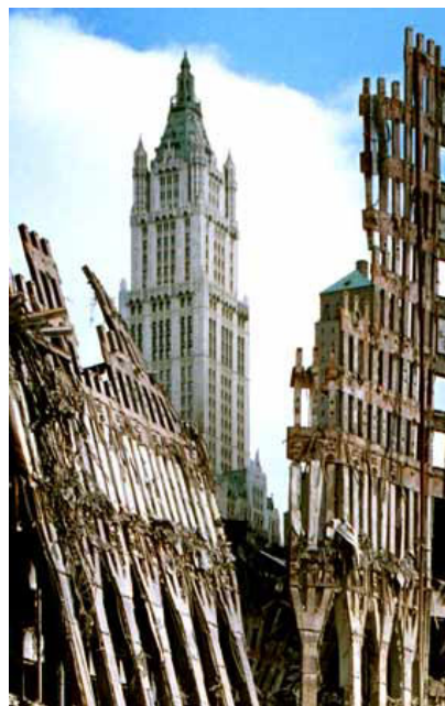
Figure 22: New York City's Woolworth Building, by Cass Gilbert, was constructed in 1913 using the Chicago Frame system. At the time of its construction in 1913, it was the world's tallest building.
