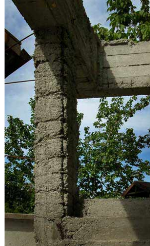
Figure 18: LEFT: House being reconstructed to replace one destroyed in Afyon earthquake. Concrete is being mixed on ground with garden hose and without slump test or measurements.
