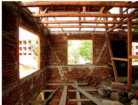
Figure 25 & 26: After witnessing the destruction of RC buildings around him in Duzce and seeing that his father's hımiş house survived undamaged, this resident of Düzce decided to stop building a new RC house and build a house for himself and his family with hımiş construction.
