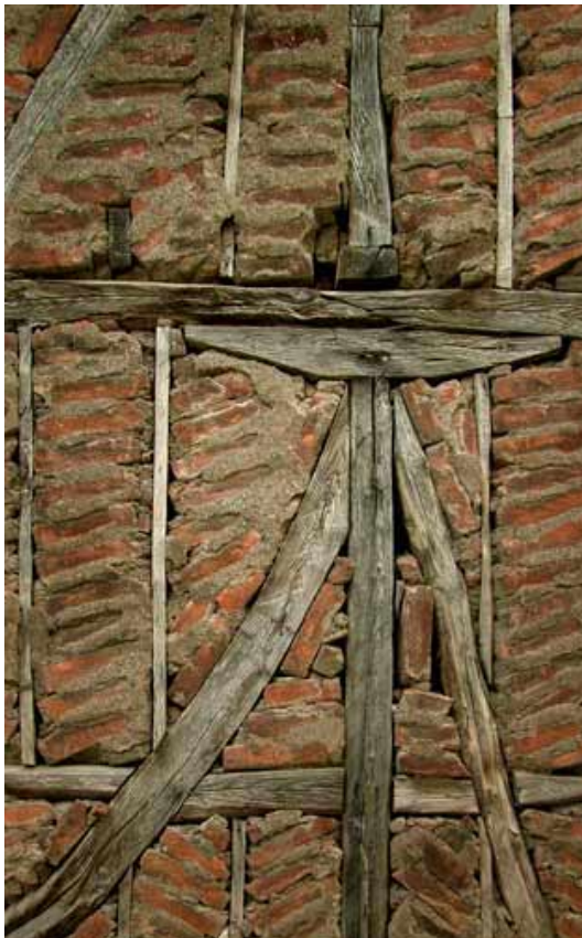
Figure 1: Hımış , traditional Turkish construction.
