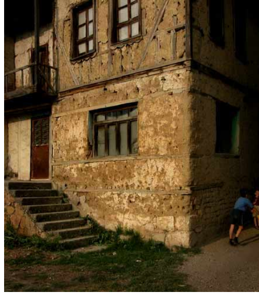
Figure 3: LEFT: Street of houses with overhanging jetties of hımış construction in Safranbolu.
