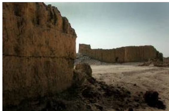
Figure 3: Unrestored ancient earthen structures including the Shahr-bast Wall in the distance after the earthquake. These structures were only lightly damaged.
