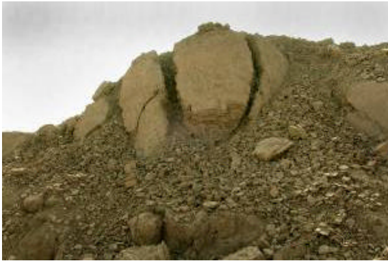
Figure 16: Collapsed round turret on the ramparts that shows evidence of having burst apart from collapse of internal layers.
