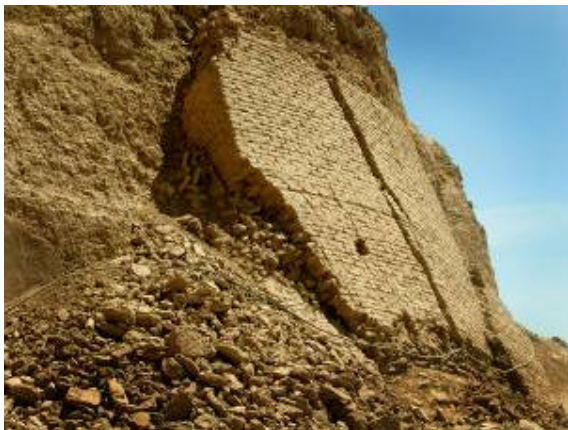
Figure 7: View of collapsed outer walls of a round tower. The Khesht construction of the outer layer has fallen off of the earlier inner layers that are most likely a combination of periods of building in different methods.
