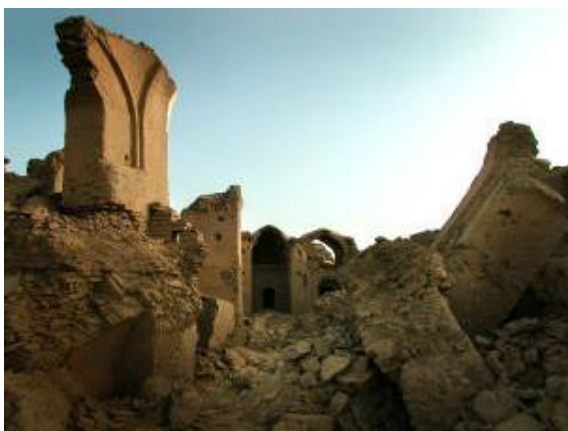
Figure 4: View of the ruins of the Arg-e Bam.
