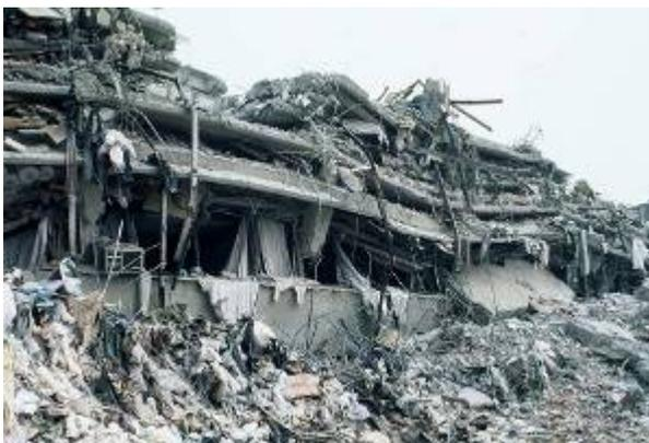
a) View of reinforced concrete (RC) Juarez Hospital in Mexico City after it was collapsed by the 1985 earthquake.
