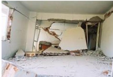
b) Typical collapsed masonry infill wall in RC multi-story residence in Gölcük, Turkey after 1999 Kocaeli earthquake.
