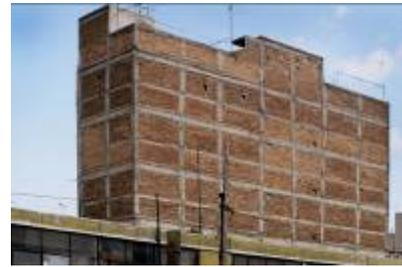
c) Building next to the collapsed Juarez Hospital (see Fig 1a) that survived undamaged. Concrete 'armature' subframes exist between the floor levels.
