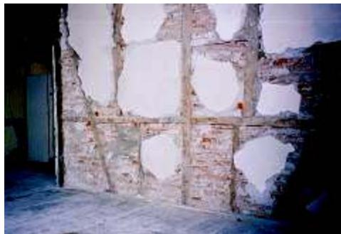
a) Masonry with timber armature *hıms* wall in Düzce, Turkey after 1999 Düzce earthquake.
