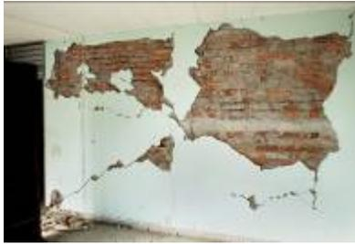
b) Upper story wall in building in (a) showing reinforced concrete sub-frame "armature" that may have prevented the collapse of upper the building's upper stories.
