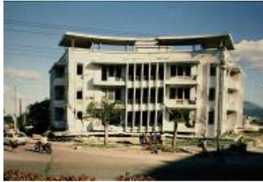
a) Apartment building after soft story collapse of ground floor during the 1987 El Salvador earthquake.
