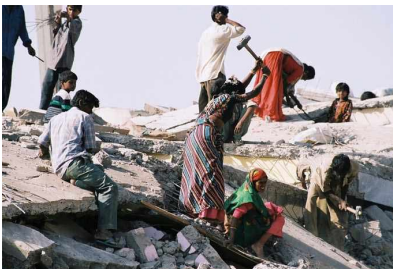
Fig.1 Demolition of collapsed RC infill building in 2001 Bhuj, India Gujarat earthquake.
