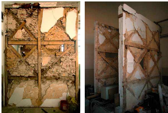
Fig.6a&b Sections from a Pombalino wall that was cut out and tested in the Portuguese Govt. lab.
