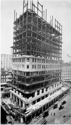
Fig.4 Flatiron Building in NYC under construction showing masonry started at 7 th floor level and at base at same time. (1901). (NY Historical Soc.)
