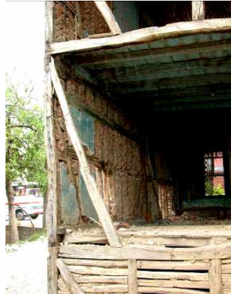
Fig.9 House in Golcuk showing humuş construction. This house was abandoned and in ruins at the time of the 1999 Kocaeli, Turkey earthquake, but remained standing with little additional damage from the earthquake
