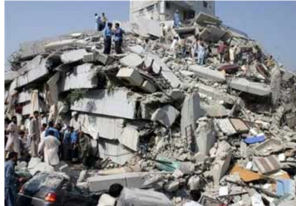
Fig.11 The Apartment tower in Islamabad that collapsed in Oct 8, 2005 was a premium project. Its failure along side other wings of the complex that survived demonstrate how hidden shortcomings in RC structures can lead to catastrophic collapse in earthquakes. Armature Crosswalls may reduce the risk of this type of collapse in such structures. (AP)
