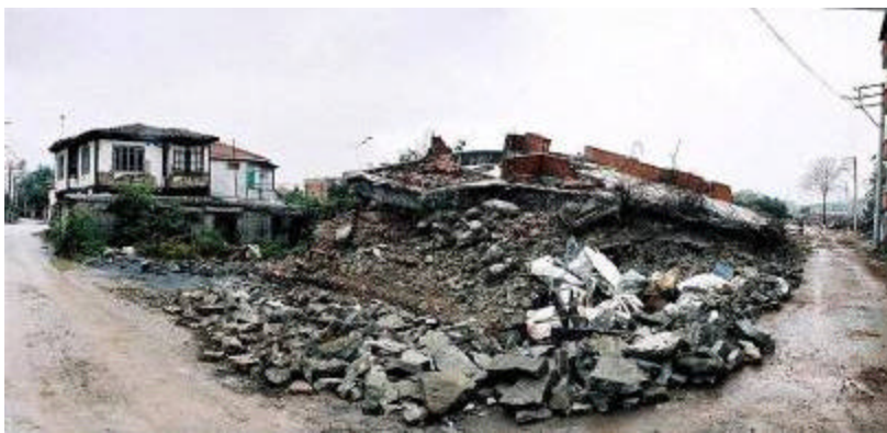
Figure 4: Surviving himis house next to a row of collapsed reinforced concrete buildings, Adapazari, Turkey, 1999.
