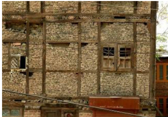
Figure 16: Example of Dhajji Dewari construction in Srinagar, 2005. The timbers form a complete frame, and the masonry is inset into the frame.
