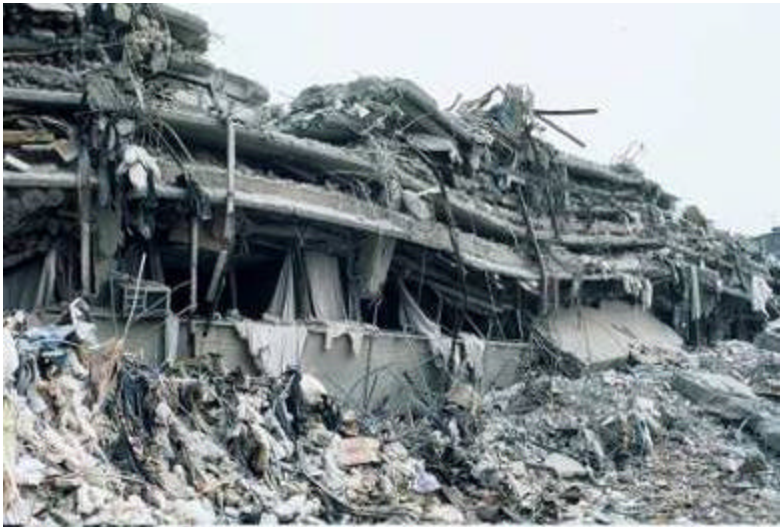
Figure 20: “Pancake” collapse in Mexico City, 1985.
