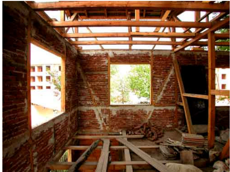
Figure 66 & 67: After witnessing the destruction of RC buildings in Duzce while his father's himis house survived undamaged, this resident of Düzce decided to stop construction of a new RC house and change it to himis construction.
