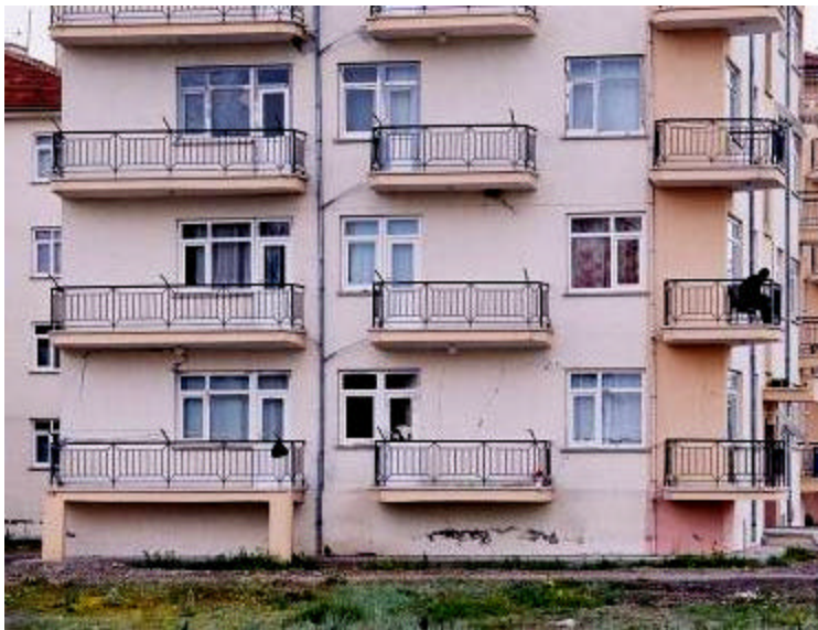
Figure 51 LEFT: RC apartment building in Orta after 2000 earthquake shows cracking in the infill walls.
