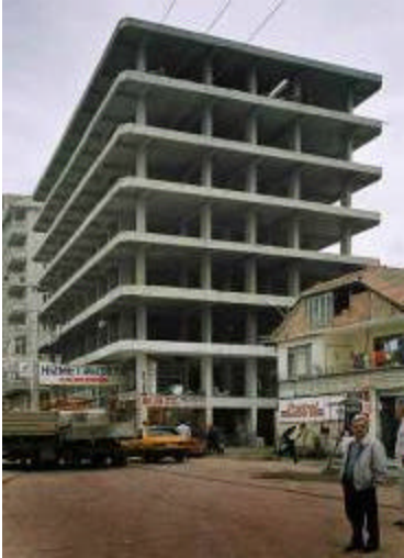
Figure 24: “Domino” frame as ideal structural form by Le Corbusier, 1915. (Giedion, 1928)
