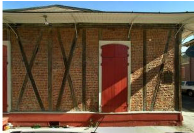
Figure 18: Colombage construction in the French Quarter of New Orleans, 2006.
