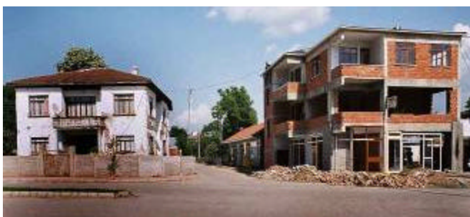
Figure 31: Three story RC building next to a 2½ story himis house near Düzce after the 1999 Düzce earthquake showing the repair of severe damage to the RC building (notice the size of the ground floor columns). The himis structure has lost only stucco on the side. Almost all of the hollow clay block on the RC building has been reconstructed after the earthquake. This shows that even low rise RC buildings sometimes suffered more damage than nearby traditional buildings.
