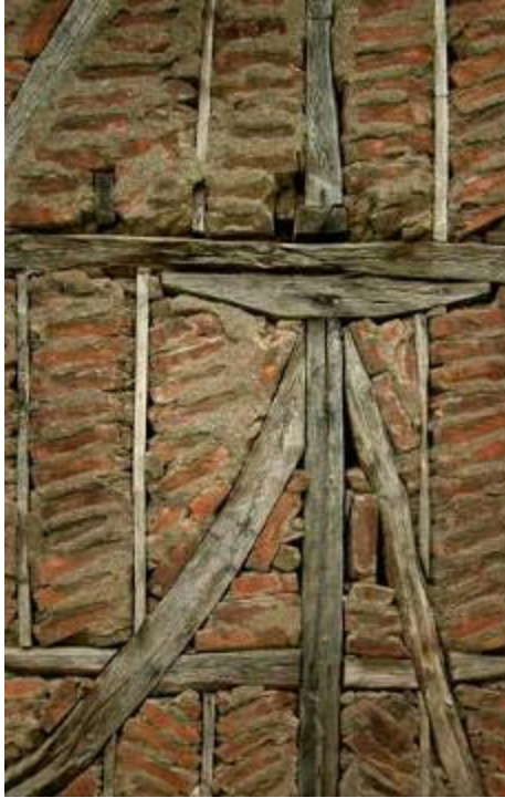
Figure 1: Detail of traditional himis construction in Turkey in mid-20 th century house in Gölcük.
