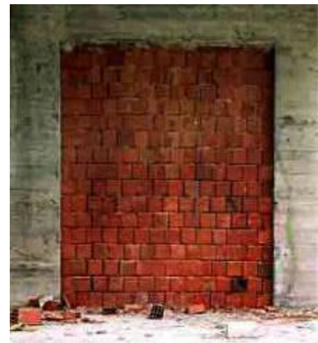
Figure 23: Typical hollow clay block infill as used in reinforced concrete residential construction in Turkey.
