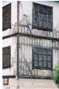
Figure 43: Large 3 story house in himis construction, Safranbolu, Turkey, 2000. Safranbolu is now on the World Heritage List because of its unique collection of intact Turkish vernacular houses.
