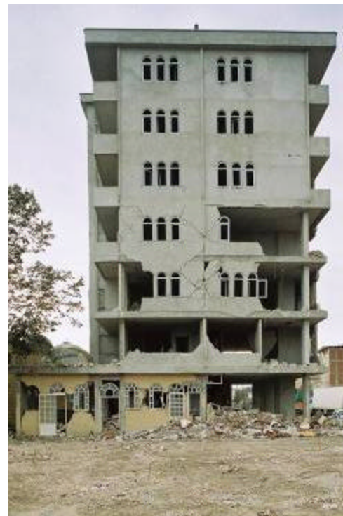
Figure 51 LEFT: RC apartment building in Orta after 2000 earthquake shows cracking in the infill walls.
