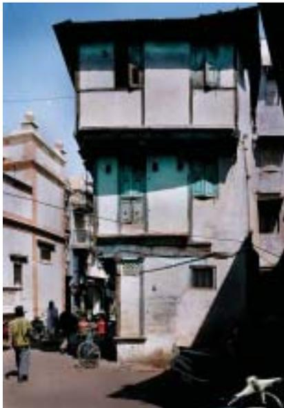
**Figure 22.** Timber-laced masonry building in Ahmedabad historic walled city area undamaged by earthquake © Randolph Langenbach, 2007.
