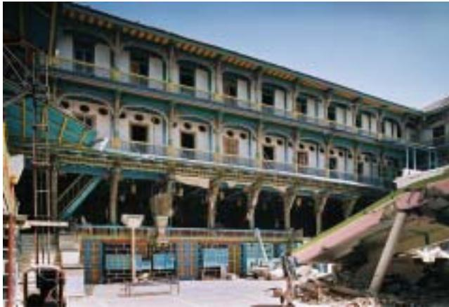
**Figure 21.** Timber-laced masonry Swaminarayan Temple in Bhuj, India, undamaged by the earthquake that collapsed the modern concrete structure in foreground. © Randolph Langenbach, 2007.
