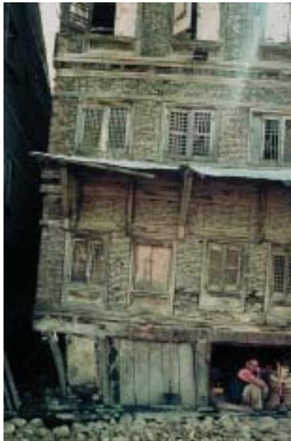
**Figure 4.** Old canal-side warehouse of *Taq* construction, Srinagar, Kashmir, India. 1981. © Randolph Langenbach, 2007.
