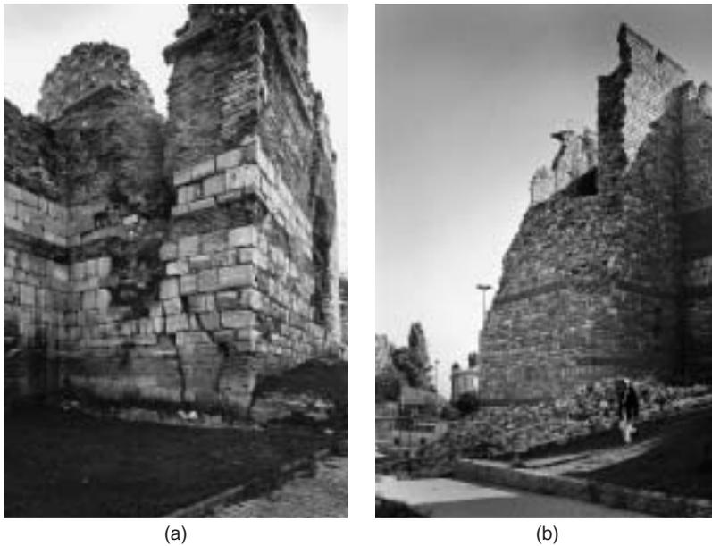
**Figure 8.** (a) Deteriorated original section of the Theodosian City Wall, Istanbul, Turkey, after the 1999 earthquake. The earthquake caused none of this damage. © Randolph Langenbach, 2007. (b) Reconstructed section in 1999 of the Theodosian City Wall Istanbul, Turkey, that collapsed during 1999 earthquake. The bands of brick, which had originally penetrated the wall, were treated as a veneer in the reconstruction. © Randolph Langenbach, 2007.
