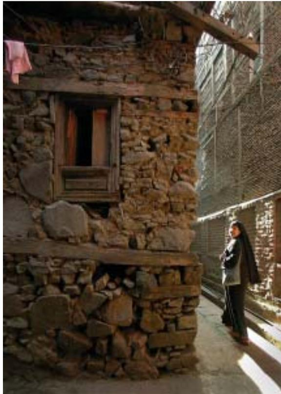
**Figure 34.** An historic house of *Taq* construction still extant in Srinagar, Kashmir, India in 2005. Rather than serving to as a condemnation, the good performance of traditional timber-laced construction in the damage district of the October 2005 earthquake should serve as an inspiration for the preservation of these often unrecognized, but rich cultural artifacts. © Randolph Langenbach, 2007.
