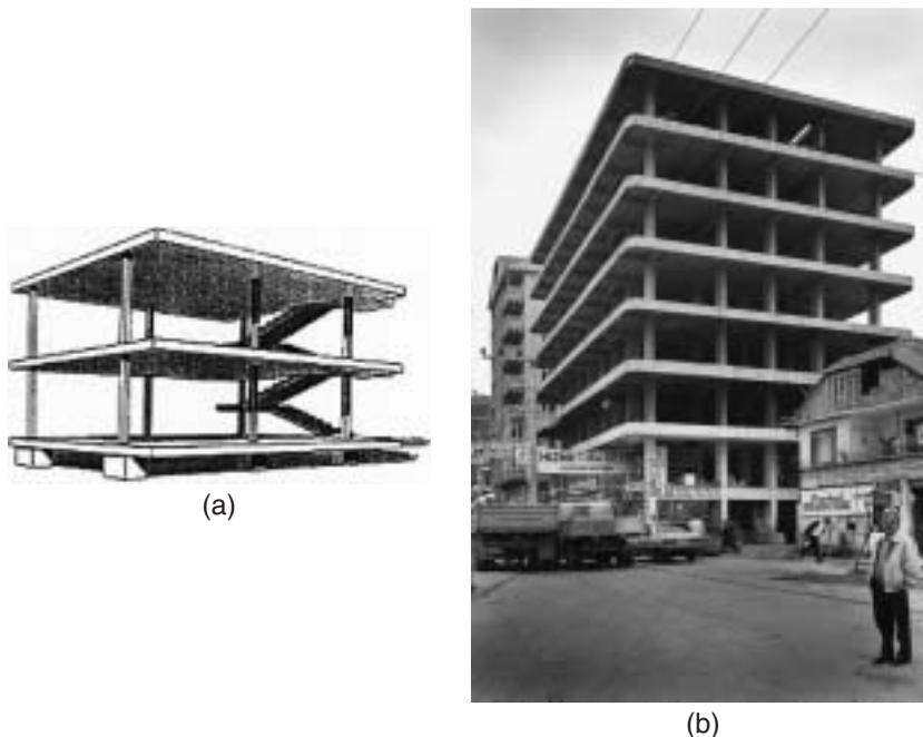
**Figure 30.** (a) Le Corbusier's conceptual Dom-Ino House, 1915 (Giedion, 1941). (b) Building under construction in Gölcük, Turkey, at the time of the 1999 earthquake. (Reinforced concrete buildings that had not been finished with the infill masonry at the time of the earthquake were much more likely to survive without collapse.) © Randolph Langenbach, 2007.
