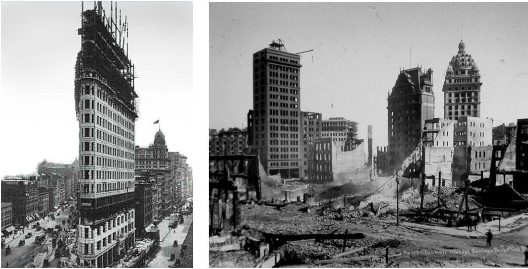
Figure 10. left: Flatiron Building in New York City under construction in 1902 showing the heavy stone masonry façade resting on the steel frame. The upper walls are constructed separately probably to ensure the weight is bearing on the frame rather than the lower masonry walls. Credit: vazyvite.com. right: View of San Francisco after the 1906 earthquake and fire. The three tall buildings visible in this view were burned out by the fire that followed the earthquake, but all three were in good enough condition despite this to be repaired, and they are still extant today. Credit: Bancroft Library.
