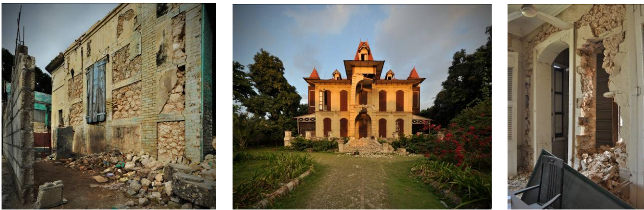
Figure 6. left: masonry wall in Port-au-Prince after the earthquake showing the typical Haitian construction with brick surrounding panels of rubble stone. middle: The Villa Castel Fleuri, a mansion in the Gingerbread District of Port-au-Prince after the earthquake. right: Interior of Villa Castel Fleuri showing partial collapse of a rubble masonry panel between the brick piers.
