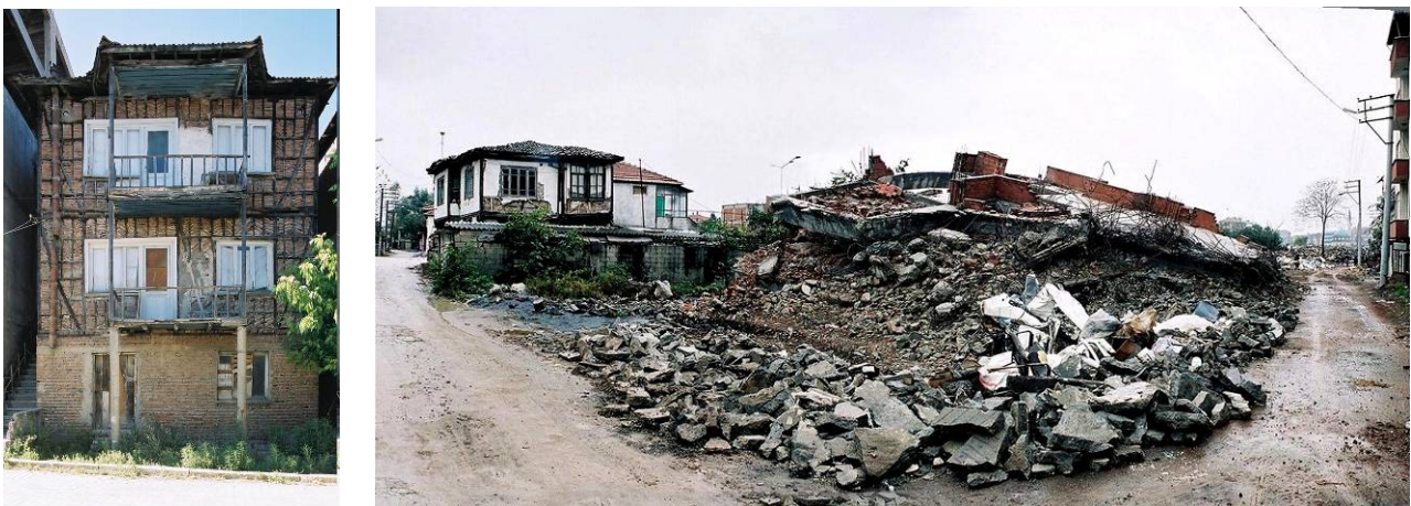
Figure 3. left: Undamaged three story himiş house in Gocuk, Turkey after the 1999 earthquake. right: View of a collapsed row of reinforced concrete apartment buildings with himiş house standing behind.
