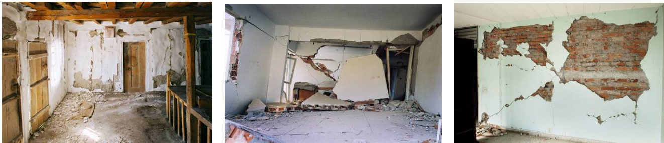
Figure 12. left: Interior of a traditional house in Yuva, Turkey of after the 2000 Orta earthquake showing evidence of the working of the hımiş walls. middle: Typical hollow clay tile masonry wall in a reinforced concrete apartment building in Gölcük, Turkey collapsed by the 1999 Kocaeli earthquake. right: Typical infill masonry wall found inside the upper stories of a four story building that suffered a soft story collapse during the 1986 San Salvador earthquake showing that the infill wall was subdivided with a concrete beam and column similar to that advocated for Armature Crosswalls. These sub-frames prevented the collapse of the ground floor from progressing to a complete pancake collapse, saving the lives of the occupants.
