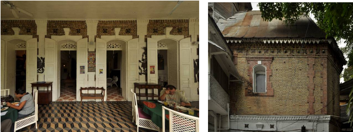
Figure 7. left: First story front wall of the Hotel Oloffson after the earthquake showing the undamaged masonry wall penetrated by many doors. right: A section of the exterior wall of the Hotel Oloffson. Most of the walls are hidden behind wide porches, but this section shows the brick construction.
