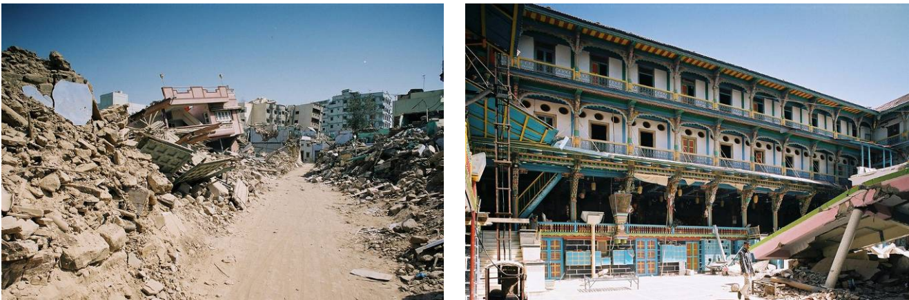
Figure 4. left: Total destruction of rubble stone and concrete buildings the city of Bhuj after the 2001 earthquake. right: Swaminarayan Temple complex in Bhuj after the earthquake.
