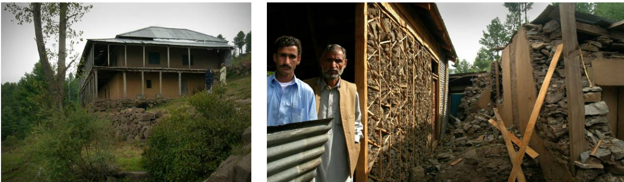
Figure 13. left: This is the only house to survive the 2005 Kashmir earthquake in the remote Pakistani village of Topi. It is of dhajji construction. right: Also in Topi, the owner (right) is standing next to his carpenter in the half-completed dhajji house he was building next to the ruins of the rubble stone house that collapsed in the earthquake seen on the right. He is using dhajji after seeing that the house on the left is the only one that survived. By proceeding with dhajji for his reconstruction, the owner was forgoing government disaster assistance which mandated using their reinforced concrete specifications. One year after the earthquake, shortly after this picture was taken, the government approved dhajji construction for as qualifying for disaster assistance. [16]
