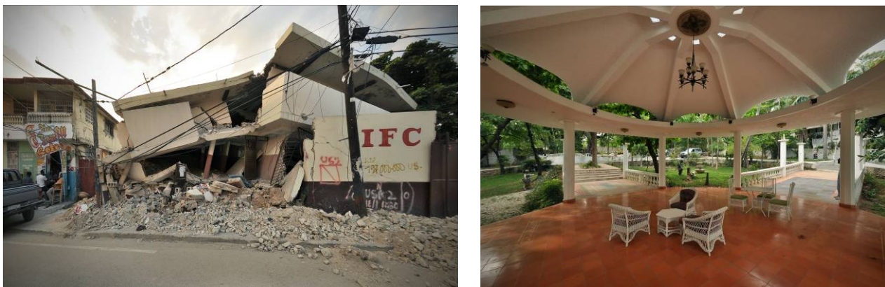
Figure 9. left: An example of vulnerable construction: earthquake collapsed reinforced concrete building, Port-au-Prince. right: An example of good construction: view of large open air gazebo at the Hotel Oloffson of reinforced concrete construction that survived the earthquake with nothing more than a few cracks in the pantry wing behind the photographer.
