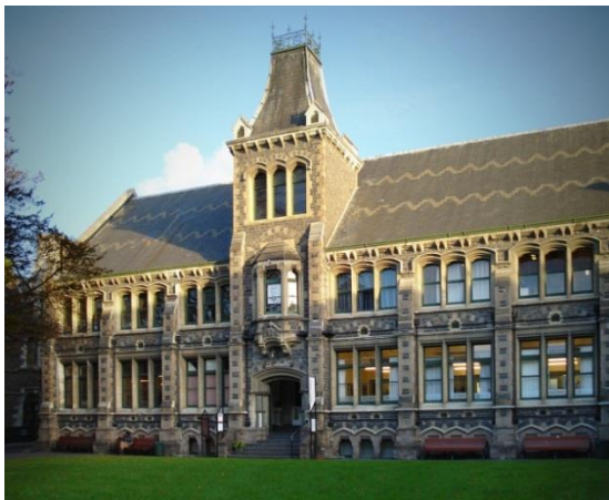
Figure 21. Chemistry block of the former Canterbury University Campus (now “Arts Complex”) in Christchurch viewed before the earthquake. Only the top of the central tower was significantly damaged in the earthquake while other unretrofitted buildings around it were collapsed.
