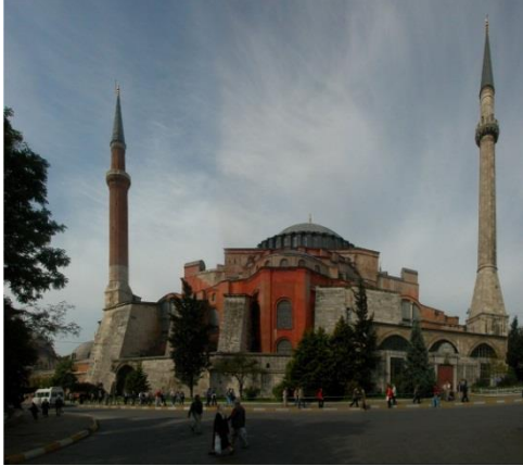
Figure 3. The Hagia Sophia in Istanbul has existed for over one and a half millennia. Repairs have been done and buttresses added after repeated earthquakes.
