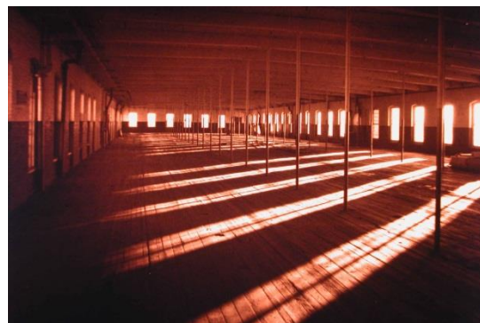
Figure 2. Interior of Mill showing typical “slow burning” heavy timber construction and brick masonry walls, Amoskeag Millyard, Manchester, NH, USA, Ca. 1835.
