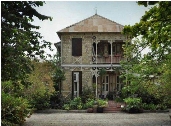
Figure 27. This house of colombage construction was in the heart of the 2010 Haiti earthquake damage district in Port-au-Prince. It suffered only minor damage while many RC buildings less than a quarter of its age collapsed on nearby lots around it.
