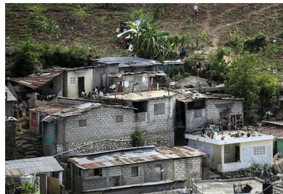
Figure 18. Typical view of informal slum houses of low quality concrete block confined masonry that survived largely undamaged, photographed in Port-au-Prince, Haiti after the 2010 earthquake. Photo, Carlos Barria, Reuters.
