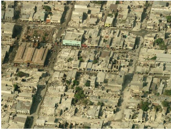
Figure 15. Aerial view of downtown Port-au-Prince after the 2010 Haiti earthquake showing the widespread numbers of collapsed buildings. Oblique aerial photographs done by Pictometry International Corporation.
