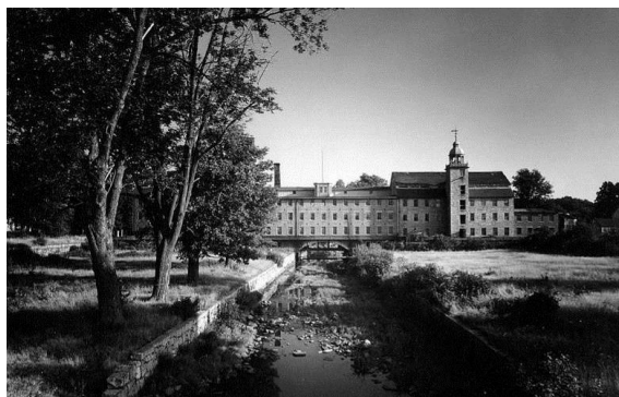
Figure 1. Crown and Eagle Mill, Uxbridge, MA., USA, ca. 1825. All Photographs in paper by © Randolph Langenbach, 2013 except when marked.
