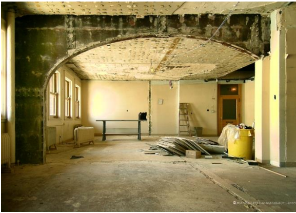
Figure 23. Portal frame arch in 1891 steel frame addition to Monadnock Building showing an element of design prior to use of contraflexure methodology.
