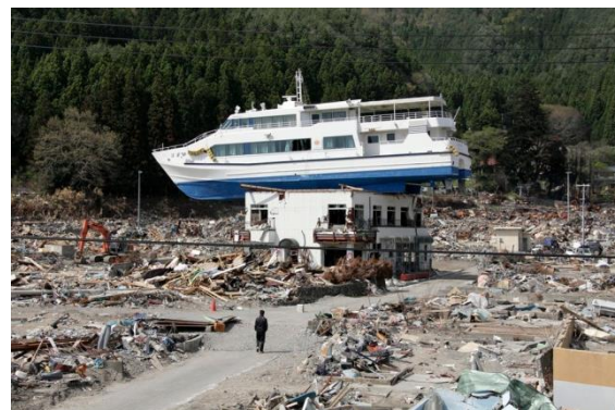
Figure 8. A boat on the roof of the only surviving building in this view in Otsuchi, Japan after the 2011 Tsunami demonstrates the remarkable resilience a well-constructed RC building. Photo: Kimimasa Mayama/EPA published by the Boston Globe.
