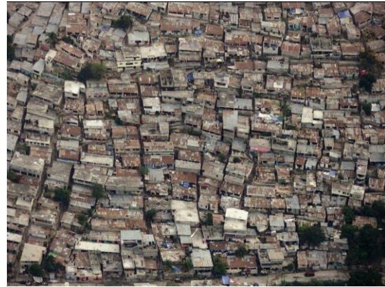
Figure 16. Aerial view of informal slum settlement near central Port-au-Prince showing slum housing that is almost entirely still standing after the earthquake. This was typical for most of these settlements except for those areas on steep slopes. Photo: Pictometry International Corp.
