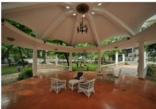
Figure 7. An RC pavilion in Port-au-Prince, Haiti after the 2010 earthquake shows that the earthquake which caused such devastation could not collapse this, in spite of the fact that it has thin columns, a heavy roof and masonry infill in only a single bay – behind the photographer.
