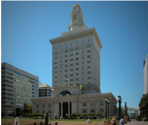
Figure 5. Oakland City Hall, Oakland, California, USA constructed in 1914. This is a steel frame, infill brick masonry building with a glazed terra cotta exterior.
