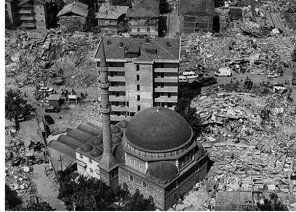
Figure 4. This intact unreinforced masonry mosque with its tall minaret in Gölcük, Turkey is surrounded by many RC buildings collapsed by the 1999 Kocaeli earthquake. Photo: Enric Marti, Associated Press
