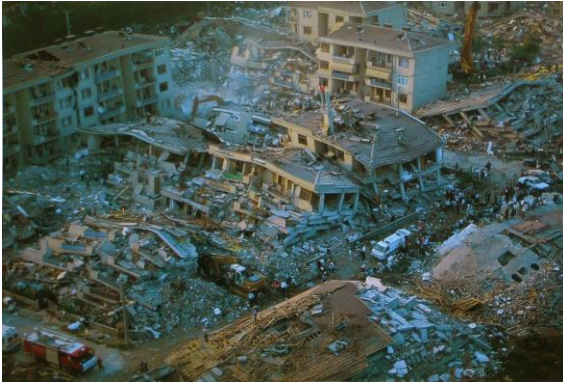
Figure 9. Aerial view of collapsed apartment houses in Golcuk, Turkey after 1999 earthquake. Most of the 17,000 fatalities (the unofficial estimate is over 25,000) in this earthquake were in pancake collapsed RC buildings. Photo UN
