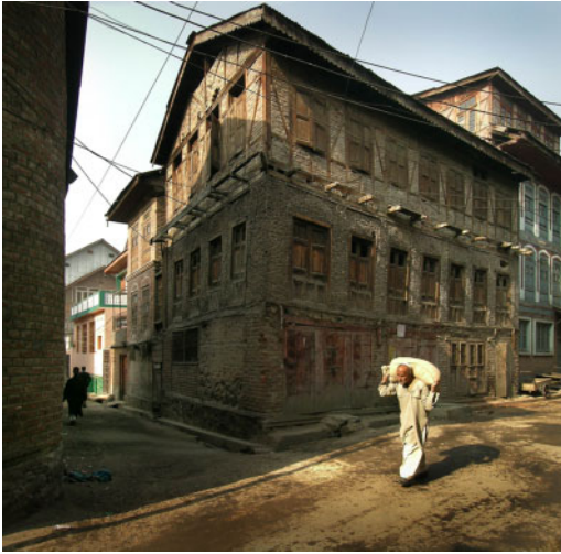
Figure 4. An older building in central Srinagar, Kashmir, India, that has taq timber-laced construction on the first two floors, and dhajji dewari infill frame construction above (Credits: Randolph Langenbach).
