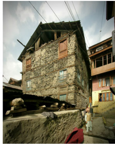
Figure 14. Four and five story residential buildings in the Indian Kashmir city of Baramulla showing how the unreinforced masonry collapsed, leaving the dhajji dewari bridging over the gap, while a tall rubble stone building reinforced with taq timber beams survived the 2005 earthquake undamaged (Credits: Randolph Langenbach).
