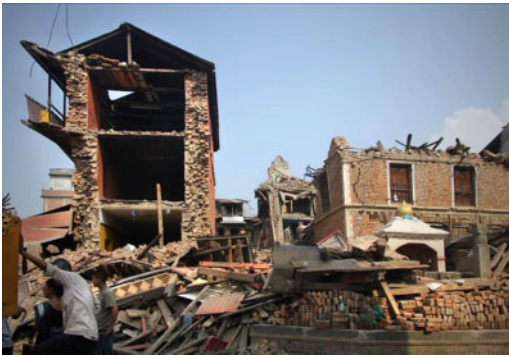
Figure 17. Unreinforced brick building collapses in Sankhu, near Kathmandu, Nepal showing the collapsed end of a row of dwellings, which lacked timber bands (Credits: Xavier Romão & Esmeralda Paupério).
