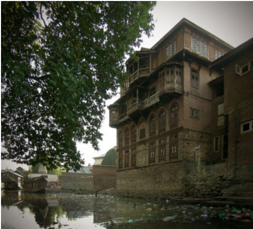
Figure 15. A grand four story bearing wall brick masonry house on the Rainawari Canal in Srinagar of timber-laced taq construction (Credits: Randolph Langenbach).
