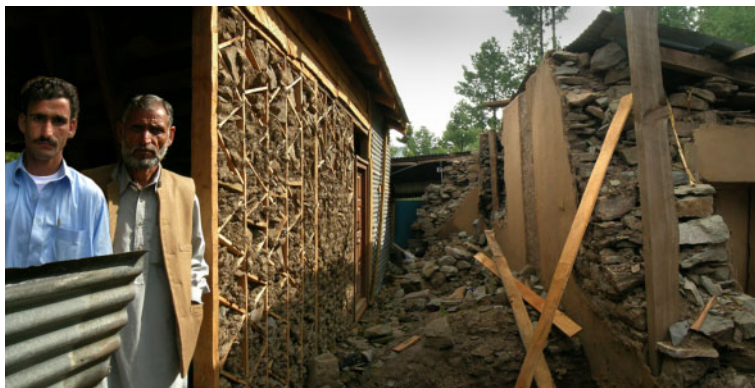
Figure 12. The owner and carpenter building a new dhajji house in Topi, near Bhag, Pakistan, to replace one of rubble stone on the right, which collapsed after seeing the survival of the building in Figure 11 and others like it (Credits: Randolph Langenbach).
