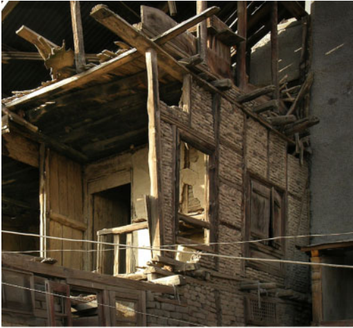
Figure 9. A cross-section of dhajji dewari construction revealed by a demolition for a road widening. Notice how thin the walls are in this form of construction. Despite this, it has proved to be remarkably resilient in earthquakes. (Credits: Randolph Langenbach).
