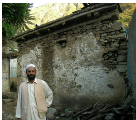
Figure 13. Villager standing near his house in a remote village between Batagram and Besham, in NWFP, Pakistan with bhatar construction which survived the earthquake. This inspired the new construction in bhatar seen on right (Credits: Randolph Langenbach).
