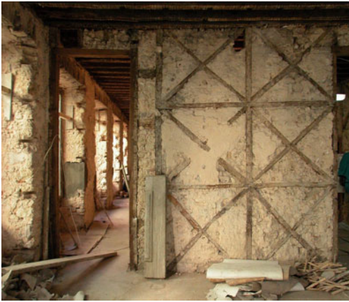
Figure 19. Interior of post-1755 Lisbon, Portugal, earthquake building in Baixa, Lisbon with interior walls of gaiola exposed during a remodeling (Credits: Randolph Langenbach).
