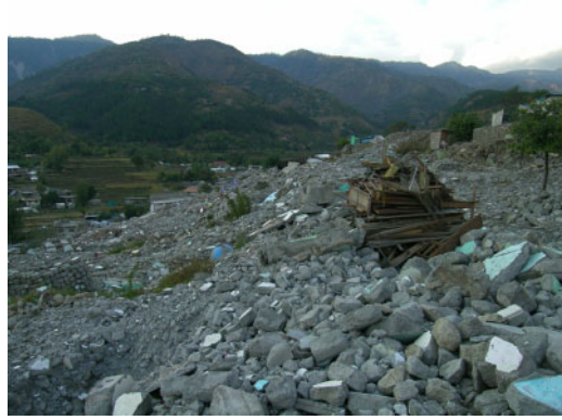
Figure 10. The debris left from the total collapse of almost all of the concrete slab and stone walled houses in Balakot, Pakistan in the 2005 earthquake (Credits: Randolph Langenbach).
