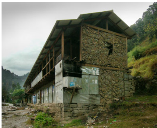
Figure 11. Country store of dhajji construction in Pakistan Kashmir near the epicenter of the 2005 earthquake. This and other buildings like it are what the local residents saw that inspired them to rebuild dhajji houses (Credits: Randolph Langenbach).
