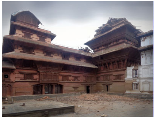
Figure 18. Hanuman Dhoka Palace, Kathmandu after the earthquake showing a section with timber bands – visible as horizontal lines on the brick façades (Credits: Kai Weise, Kathmandu, Nepal).
