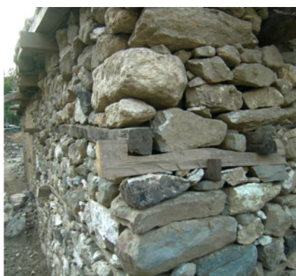
Figure 13. Villager standing near his house in a remote village between Batagram and Besham, in NWFP, Pakistan with bhatar construction which survived the earthquake. This inspired the new construction in bhatar seen on right (Credits: Randolph Langenbach).
