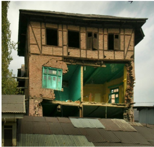
Figure 14. Four and five story residential buildings in the Indian Kashmir city of Baramulla showing how the unreinforced masonry collapsed, leaving the dhajji dewari bridging over the gap, while a tall rubble stone building reinforced with taq timber beams survived the 2005 earthquake undamaged (Credits: Randolph Langenbach).
