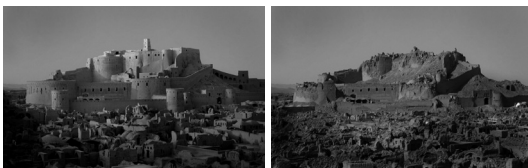
Fig. 4. Arg-e-Bam, before and after 2003 quake. (left photo courtesy of Kerman Province).
