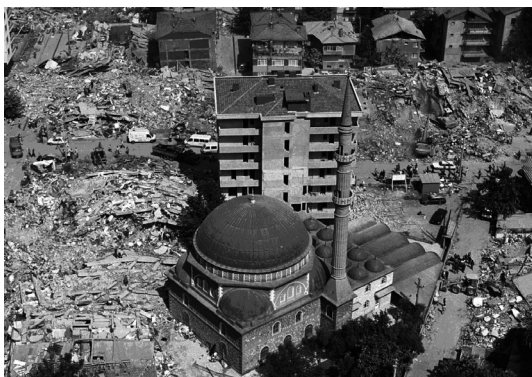
Fig. 1. Gölcük, Turkey after 1999 Kocaeli earthquake. (AP photo by Enric Marti (NY Times, Aug.20, 1999.)
