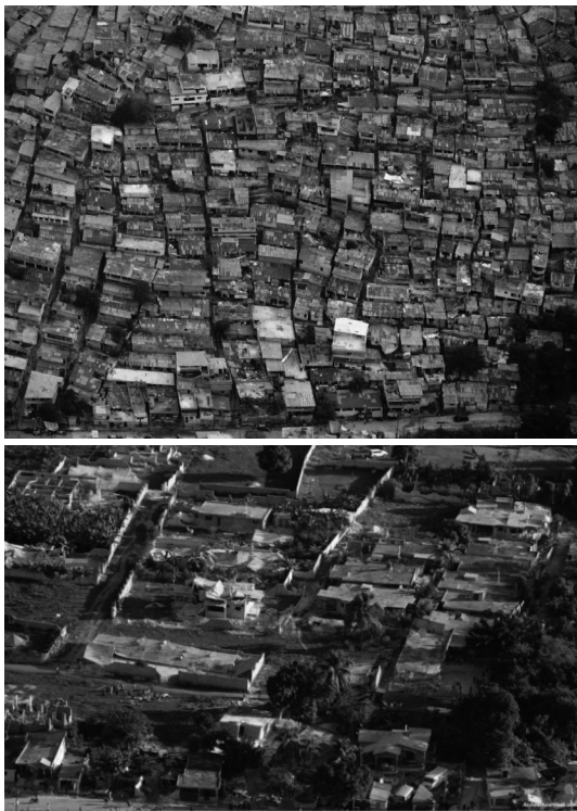
Fig. 6. Pictometry Int'l Corp photos of slum settlement (bidonville), and (bottom) upper-class houses, after 2010 earthquake.
