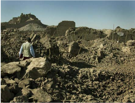
Figure 1.2 Earthquake destruction of the restored parts of the Arg-e-Bam photographed four months after the earthquake.
