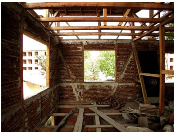
Figure 1.29 The interior of the new house being constructed by this family shown in Figs. 1.27 and 1.28 being built of traditional Turkish humuş construction.
