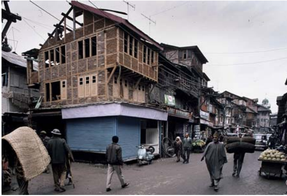
Figure 1.18 New construction in dhajji-dewari photographed in 1989. More recently, this form of construction has largely gone out of use, in favor of reinforced concrete.
