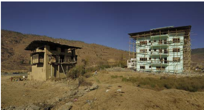
Figure 1.6 New construction in reinforced concrete next to a traditional earthen house near Thimphu, Bhutan, 2010.
