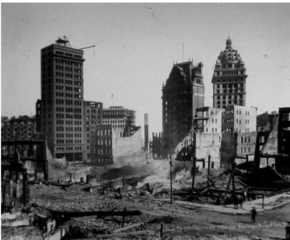
Figure 1.19 View of San Francisco showing three of the steel skeleton frame buildings after the fire had burned them out. These included the 315 foot high steel skeleton frame Call Building constructed in 1890. All of the surrounding buildings, except for the skeleton frame structures, were completely destroyed. These three skeleton frame structures, as well as most of the others in the city from that time, were repaired and about half of them still exist today.
