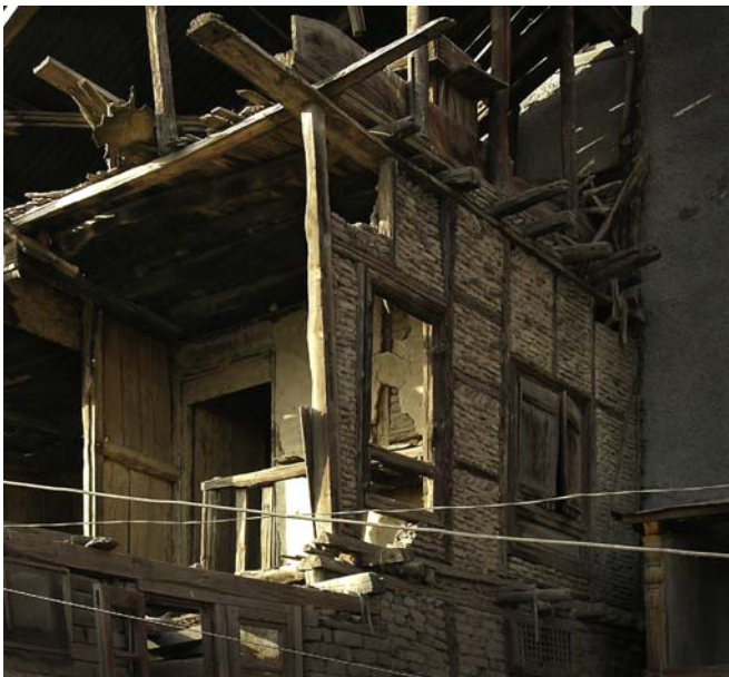
Figure 1.17 Dhajji-dewari building showing the single-leaf construction of the walls. The building was under demolition for a road widening, 2005.
