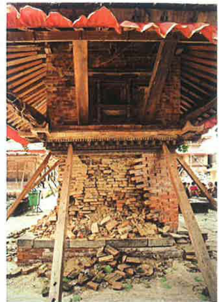
11-12/ Small pagoda temple in Kathmandu Durbar Square which almost was toppled by the earthquake, showing the shedding of the wedge shaped face bricks which lack bond courses and bow outwards when compressed during an earthquake.
