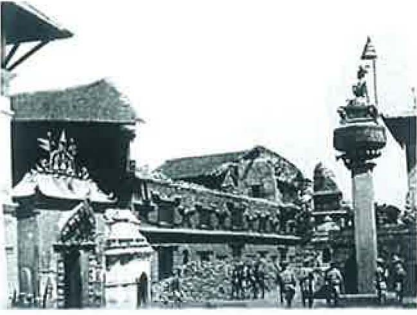
5-6-7 / Fifty-five Windows Palace (18th century), Bhaktapur, after the 1934 quake (6a); in year 2000 (6b) showing tilted and deteriorated front brick wall with the windows after being rebuilt without their historic projection after the 1934 earthquake, but prior to the full restoration in 2005; view after the 2015 earthquake (6c) showing no damage. Photo's source: Images of a Century, Editor: Andreas Proksch, Deutsche Gesellschaft für Technische Zusammenarbeit (GTZ) GmbH, 1995
