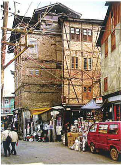
3/Srinagar; Kashmir showing taq on left, and dhajji dewari on right.
