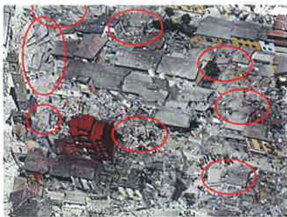
II Amatrice after the 24th August 2016 earthquake showing evidence of reinforced concrete slabs in debris (AP photo).
