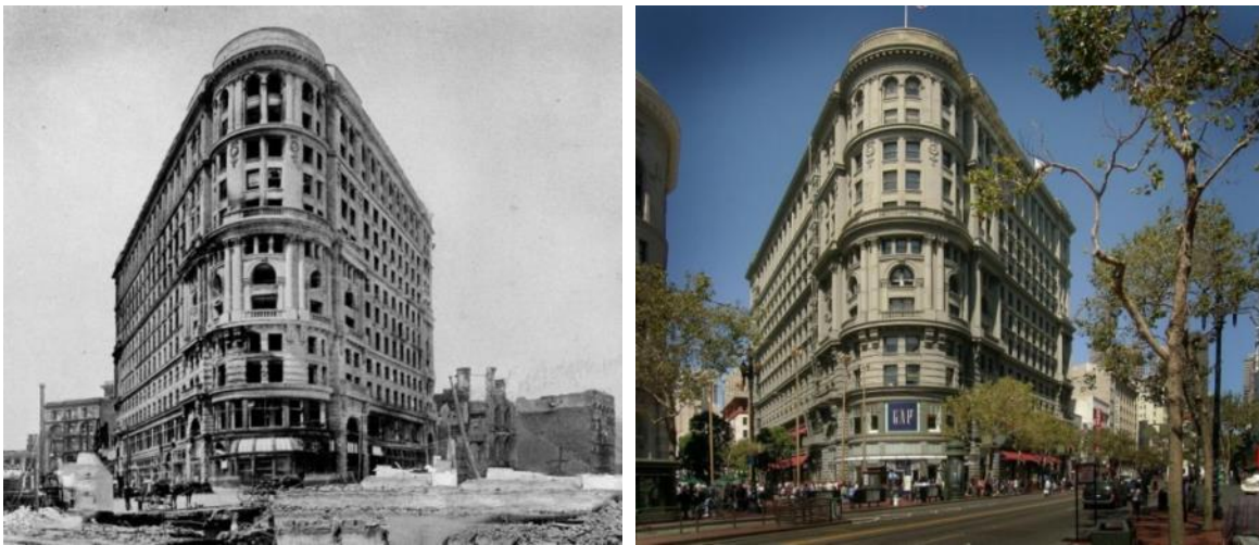
Figure 34: The Flood Building, San Francisco, constructed in 1904, It is twelve stories with a steel frame and thick infill masonry. (Left) after the Great 1906 earthquake and fire, and (right) its appearance today. It was simply repaired from the earthquake and fire damage after the earthquake. It did not have to be rebuilt.
