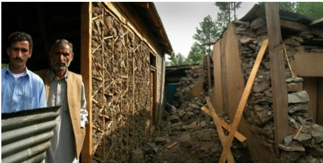
Figure 6: New dhajji next to ruins of URM house
