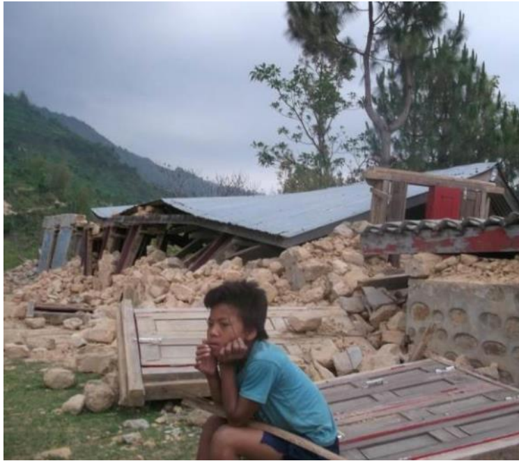
Figure 56: School building totally collapsed in 2015 Ghorka Earthquake with sheet metal roof.
