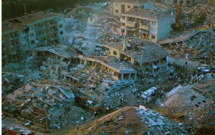
Figure 35: Collapsed RC Buildings in Gölcük, Turkey after 1999 Kocaeli earthquake
