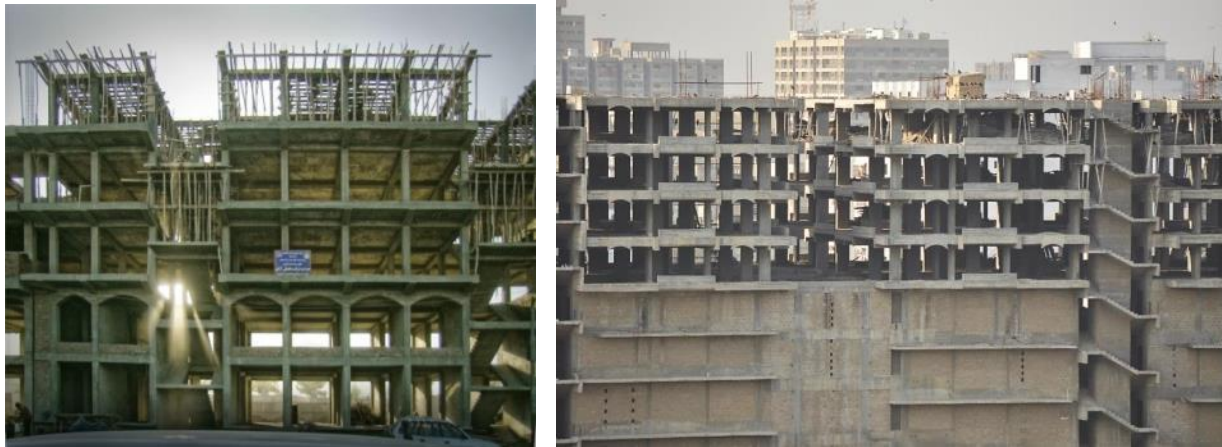
Figure 30: 5+ story RC moment frame building under construction in Kabul, Afghanistan
