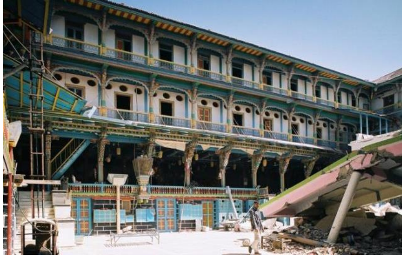
Figure 21: the Bhuj branch of the Ahmedabad-based Swaminarayan Temple, the construction is of timber frame with masonry infill which was common in Ahmedabad, but rare in Bhuj, is located in the heart of the walled city of Bhuj, yet it survived almost undamaged, while the modern concrete pavilion seen on the right collapsed
