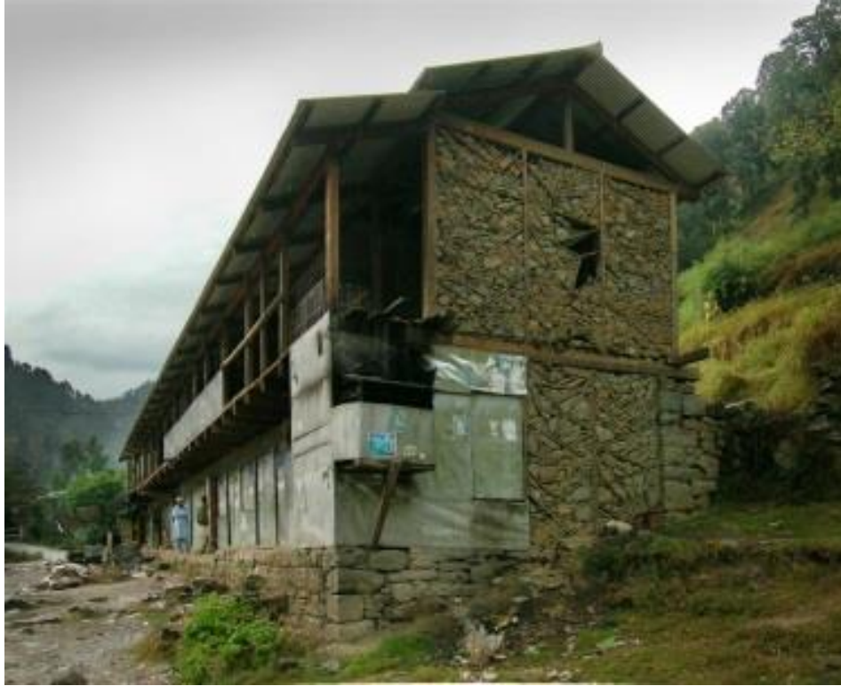
Figure 7: Large dhajji country store block on road to Thub
