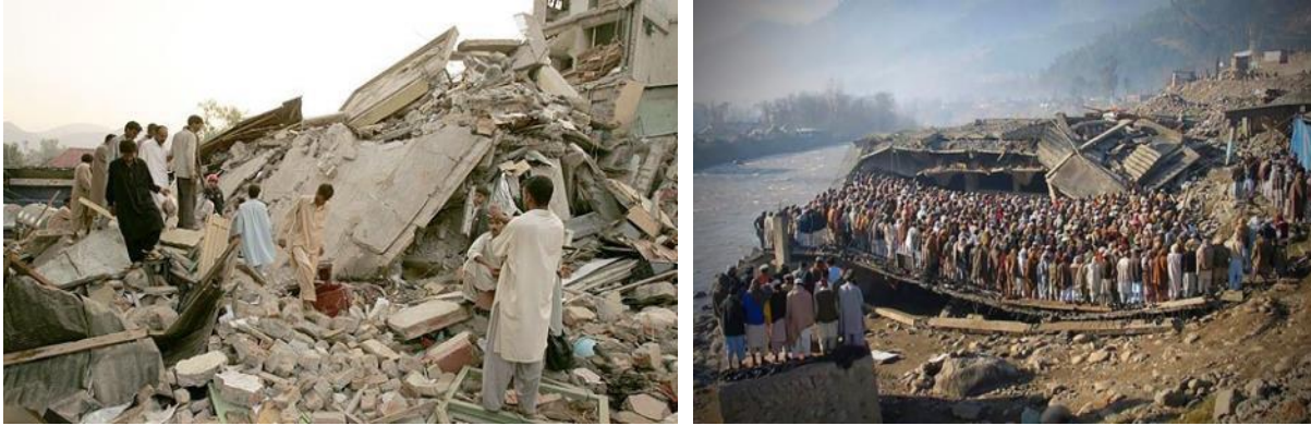
Figure 29: This is a remarkable photo taken in Balakot of an open air prayer meeting on the floor slab of the collapsed main Balakot mosque. Every building in the city was reported to have been destroyed, but the strength of this reinforced concrete floor slab to hold this many worshippers is amazing (courtesy IIEES)
