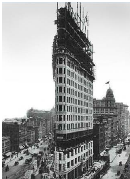
Figure 32: Flatiron Building in New York City under construction in 1902 showing the stone masonry façade resting on the steel frame. The upper walls are constructed separately from the walls below, most probably to ensure their weight is bearing on the steel frame rather than the lower masonry walls.
