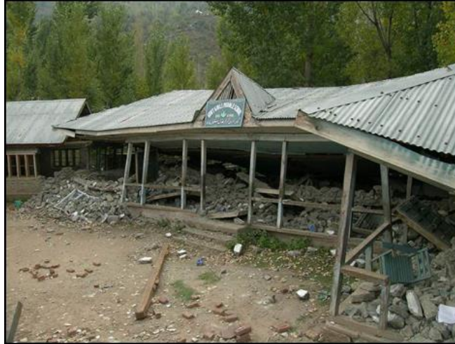
Figure 11: Collapsed School, Uri
