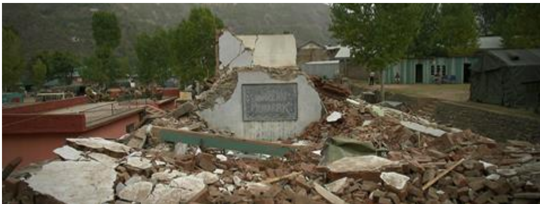
Figure 3: Collapsed School, Uri, Indian Kashmir. Written on the blackboard before the earthquake, is “ Ramazan Mubarak ” (Blessed Ramadan), which now is all that remains.
