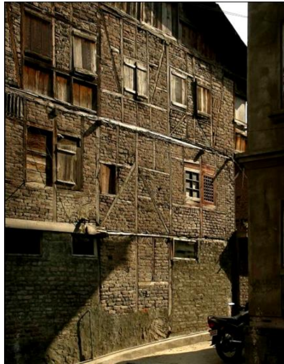
Figure 19: A dhajji dewari building in Srinagar
