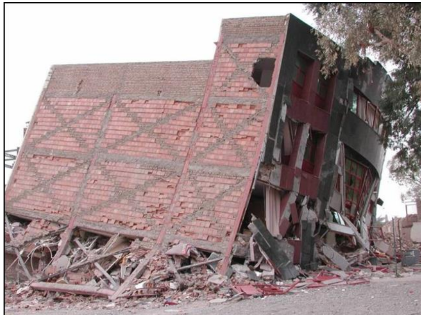
Figure 36: Collapsed steel frame building after 2003 Bam, Iran earthquake
