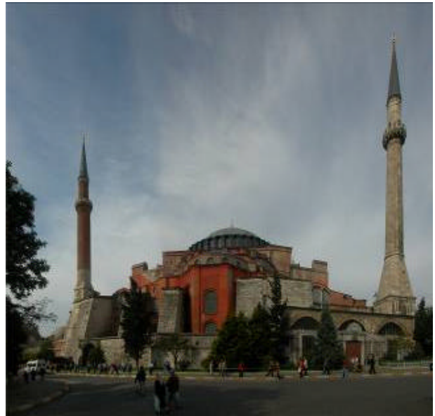
Figure 5: Exterior of the eastern side of Hagia Sophia. This view shows the many large buttresses added over the centuries to support the original church. (To be able to illustrate this view in a single image, two wide-angle photographs have been joined together.)
