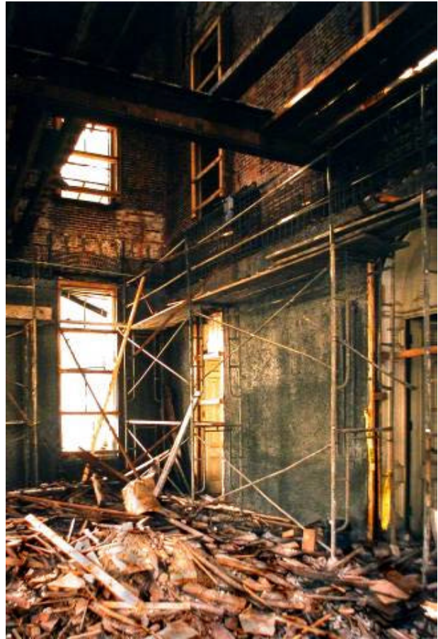
Figure 7: Interior walls of South Hall being covered by steel and shotcrete.
