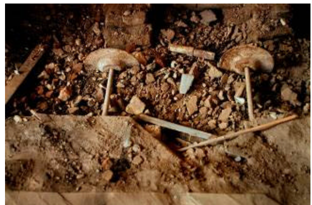
Figure 6B: Dog anchors in South Hall walls exposed by construction work.
