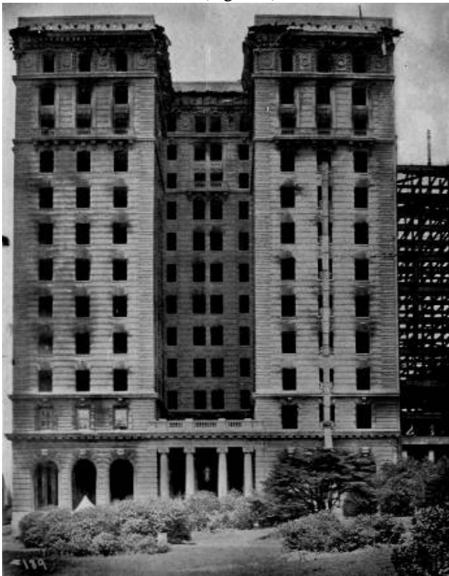
Figure 4: Burned hulk of the St. Francis Hotel in 1906. This steel frame in this building came through the fire in almost perfect condition. (FROM: A.L.A.Himmelwright, CE, The San Francisco Earthquake and Fire, The Roebling Construction Company, NY, 1906, p175.)
