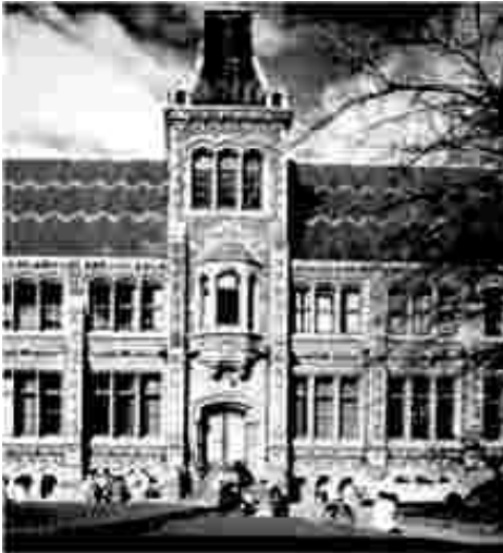
This building in New Zealand was strengthened by cables wrapped around the masonry structure. The cables function similarly to the runners in the TAO system.
