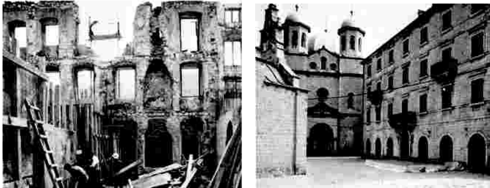
After the 1979 earthquake in Kotor Yugoslavia many buildings were completely gutted. Although the historic masonry was reattached the historic interiors have been completely destroyed
