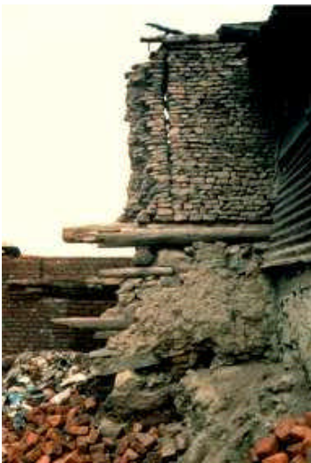
Srinagar House being demolished showing the Taq timber and masonry construction with timbers imbedded into the wall lengthwise and cross-wise.
