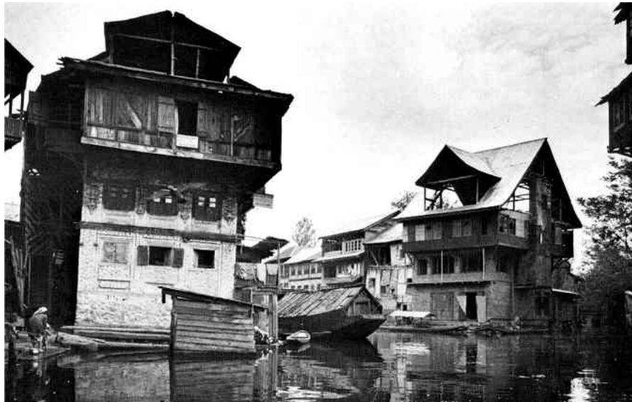
Wood and masonry houses line the Rainawari Canal in Srinagar. Many of these buildings date back to the eighteenth and nineteenth centuries, demonstrating the ability of native construction methods to withstand earthquakes.
