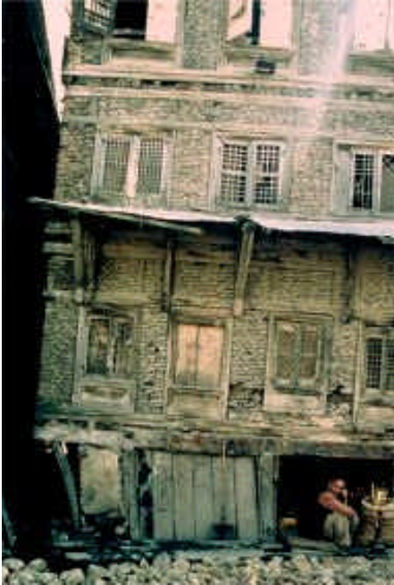
An eighteenth or early nineteenth-century canal warehouse in Srinagar illustrates the Taq system of construction. The alternating timber "runners" and brick infill create a "woven" appearance.
