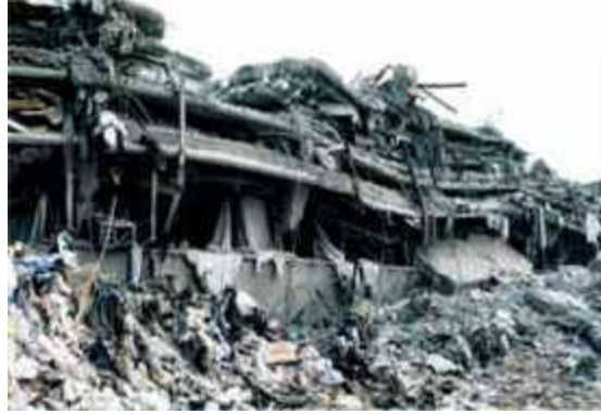
Collapsed building, Mexico City, 1995
