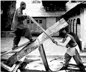
Pre-industrial building methods are still used in India. This ancient method of cutting timber into planks is not uncommon in this village in Kashmir.
