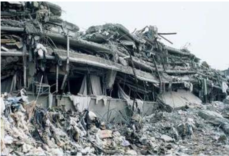
Figure 18: “Pancake” collapse in Mexico City, 1985.
