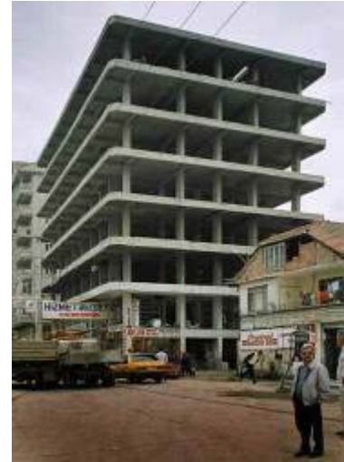
Figure 23: A massive RC frame in Golcuk, Turkey under construction at time of 1999 earthquake before installation of infill masonry walls. Much greater damage or collapse would have been likely had the infill walls been installed by the time of the earthquake.
