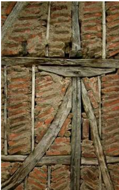
Figure 1: Detail of traditional hımış construction in Turkey in mid-20 th century house in Gölcük.
