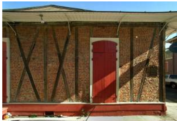
Figure 16: Colombage construction in the French Quarter of New Orleans, 2006.
