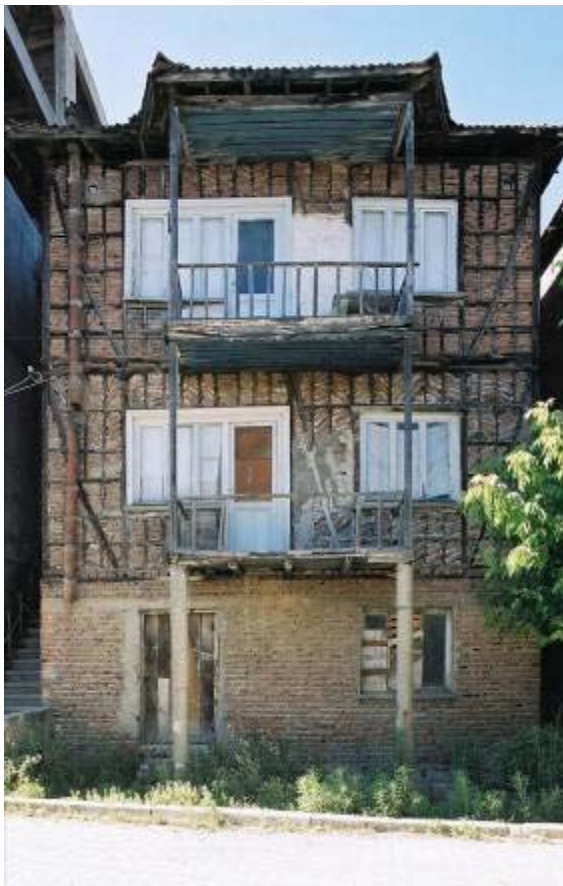
Figure 10: This three story house in Gölcük located less than one km from the fault was undamaged by the 1999 earthquake, while a number of reinforced concrete buildings on the adjacent blocks collapsed. 1
