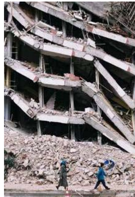
Figure 19: Partial collapse of RC Building, Gölcük , Turkey, 1999.
