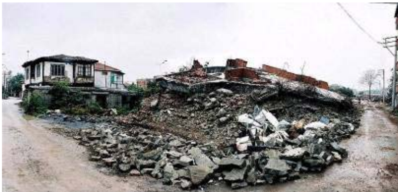
Figure 4: Surviving himiş house next to a row of collapsed reinforced concrete buildings, Adapazari, Turkey, 1999.
