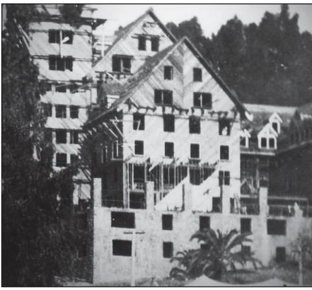
Fig. 3: Claremont Hotel under construction in 1906 (Source: University of California Berkeley Library)
